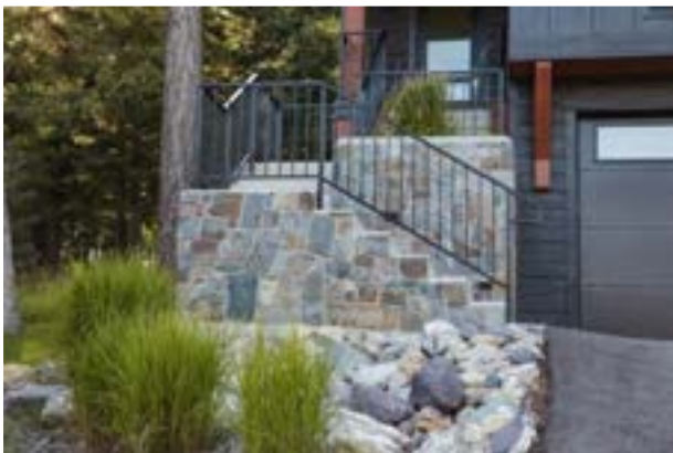
Stone cladding over concrete.
