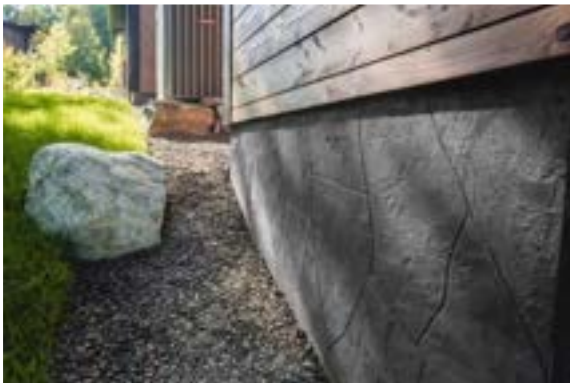
Textured architectural finish over concrete foundation.
