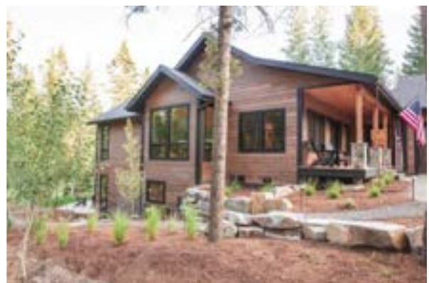
Stepped retaining wall to cover foundation.
