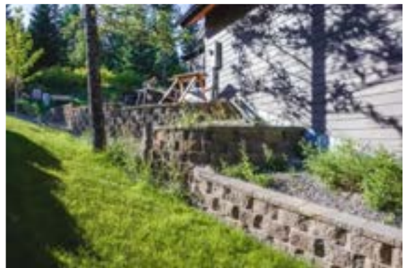
Stepped retaining wall to cover exposed foundation.
