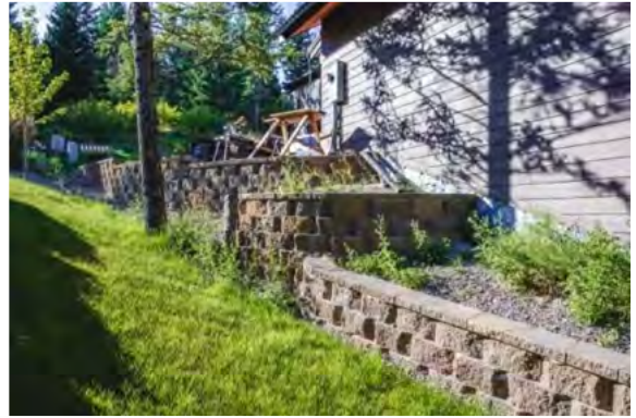
Stepped retaining wall to cover exposed foundation.
