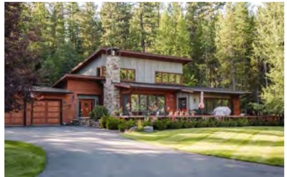
Modern style home with mono slope (shed) roof and combination of wood, metal and stone.
