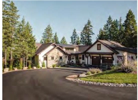
Transitional style home with gabled rooflines, shed dormer and wall masses showing architectural relief.
