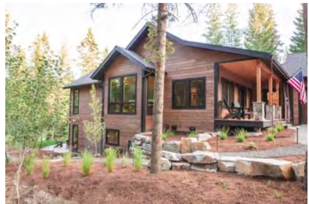
Stepped retaining wall to cover foundation.
