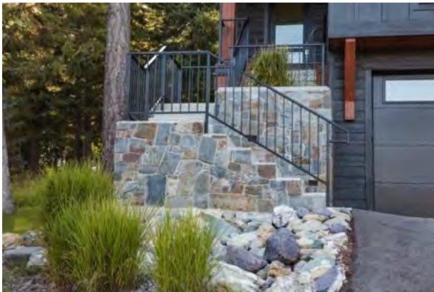
Stone cladding over concrete.
